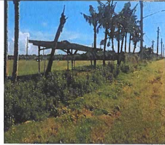
Figure 4 - Standing along Route 15, this temporary structure marks a corner of the 200' access and utilities R/W (Lot 3R/W)
